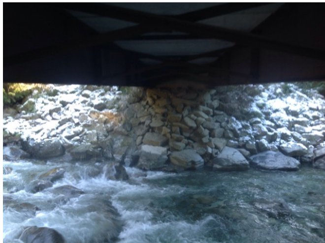
Left Bank Abutment when facing downstream
