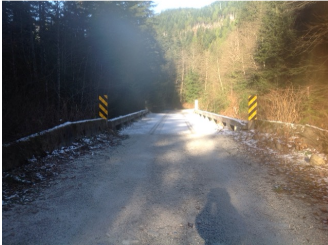
Approach from Left Bank when facing downstream
