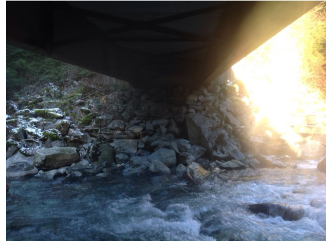
Right Bank Abutment when facing downstream
